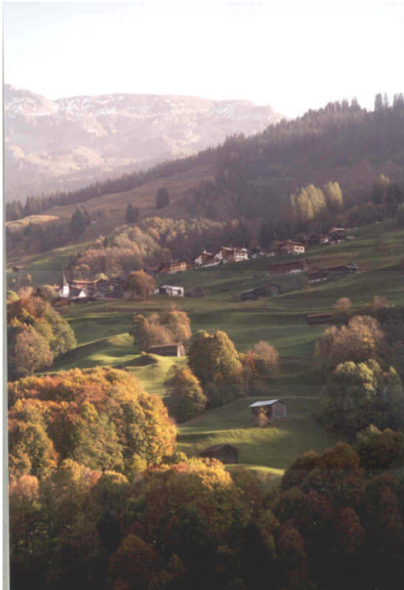
Figure 11 : The village of Conters is clearly located in a slowly moving zone of the landslide.
