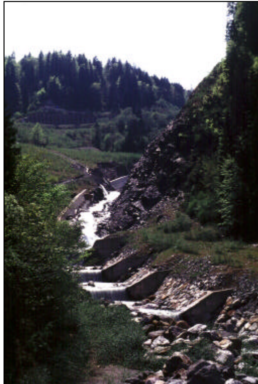
Figure 8: debris barriers and river channel
