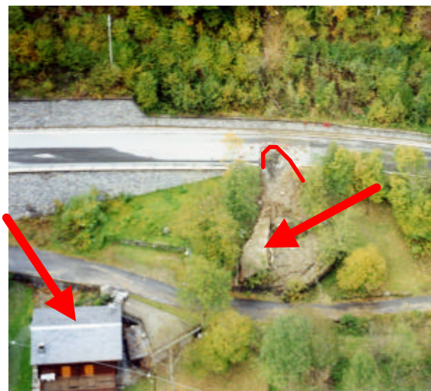
Figure 9: rock fall triggered during the October 2000 flood. The boulder (right red arrow) damaged the national road (red line) and stopped near a house (left red arrow).
